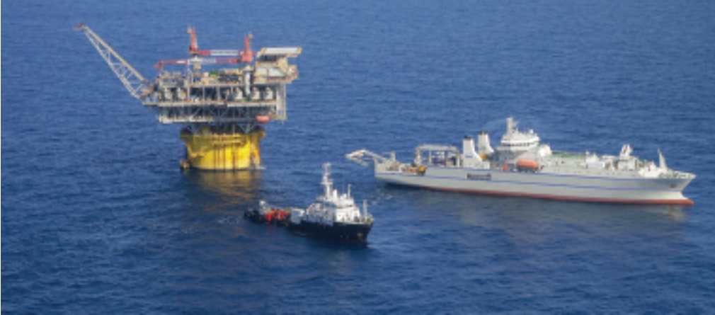
Tyco Decisive installing riser at Horn Mountain (left)
