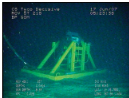
Subsea fiber optic termination utilizes wet mate connectors to facilitate system expansion
